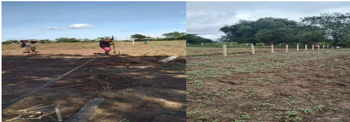
Fig. 28. Establishment of perimeter fencing in DA-Aroman, North Cotabato
