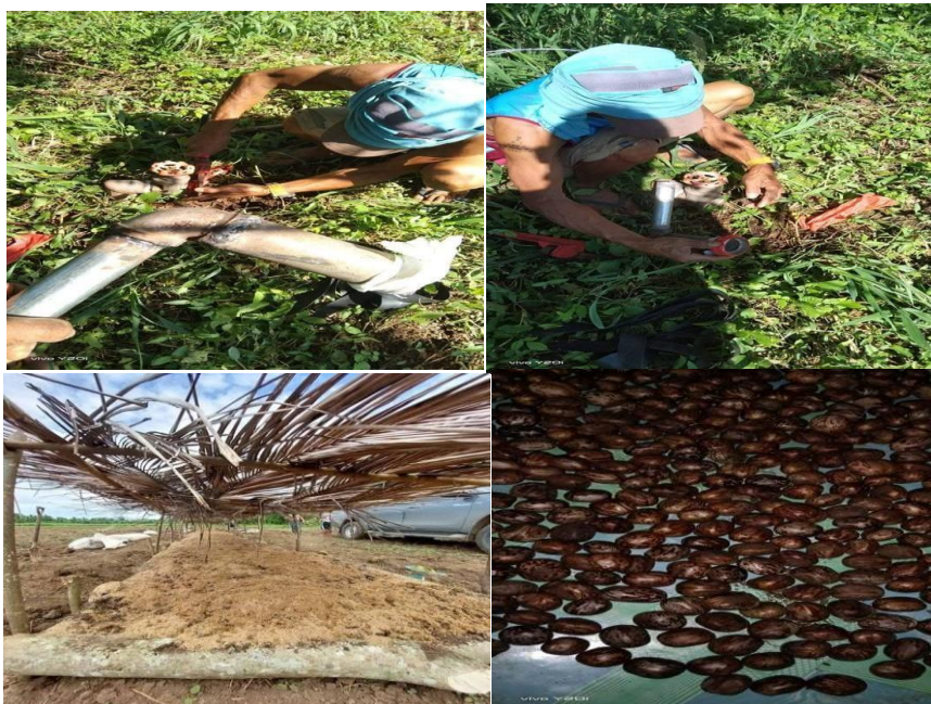
Fig. 30. Installation of Water pipe line system in DA –Aroman , North Cotabato.
