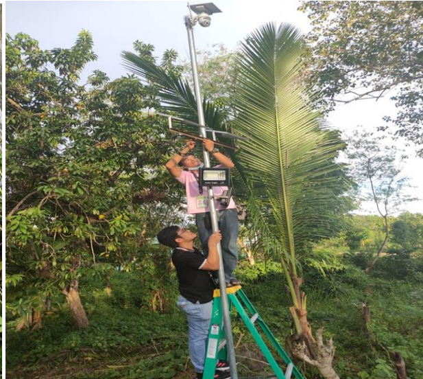
Installation of Safety Devices in the Laboratory Area
